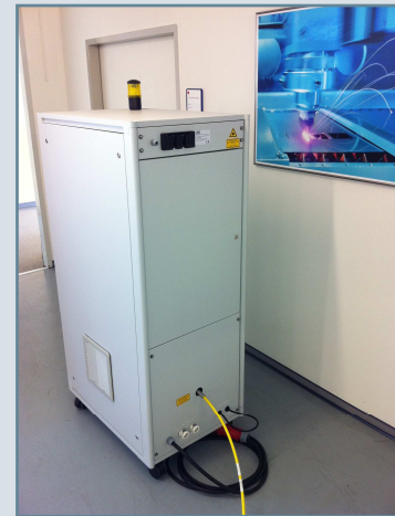
Rear view of the rack system, preliminary
